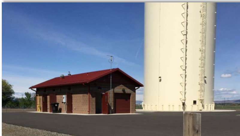
Well No. 9, its power generator, electrical room, and fluoridation/chlorination room are all within the building shown, and in separate rooms. Reservoir No. 5 is pictured here.
