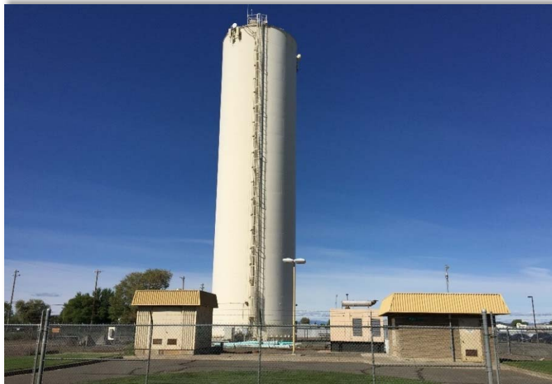
The building on the left is the well house, the building on the right is the electrical and fluoridation/chlorination building, the power generator is shown next to the electrical building, and Reservoir No. 4 is shown behind the well house.
